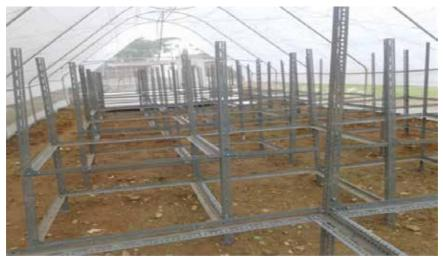
Figure 9. Construction of the aeroponics boxes frames using Dexion shelve.
