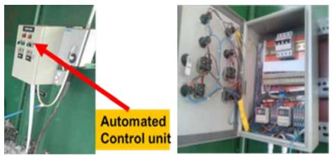
Figure 18. Automated control panel of the power house with the timers linked to the pumps.
