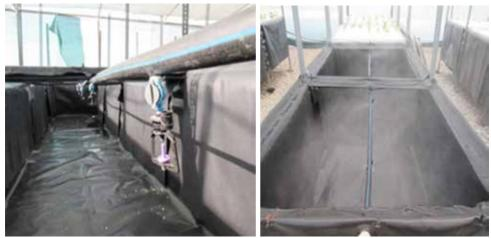
Figure 14. Picture of misters (left) and the central pipe with misters (right).
