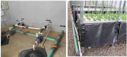
Figure 13. Piping in the power house (left) and pipes for feeding the plantlets in the boxes (right).
