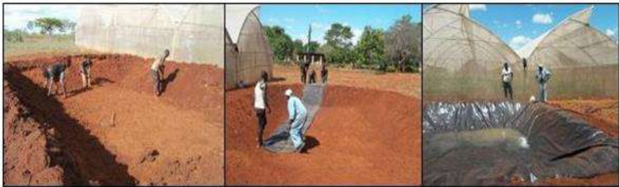
Establishing a small fishpond (left to right): 1) excavating and smoothing the pond, 2) spreading the PCV liner and burying the edges, and 3) filling the pond
