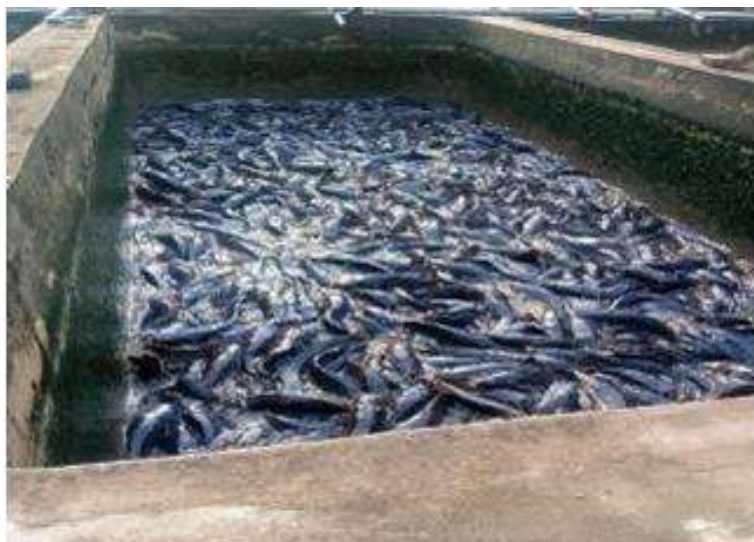
A concrete tank for raising catfish
