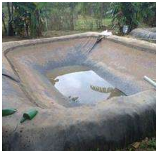
Excavated pond with liner
