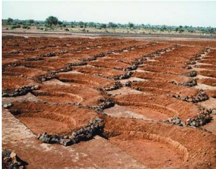
Semi-circular bunds reinforced with stones
