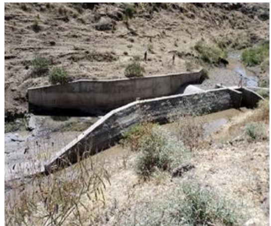
Diversion of a seasonal stream to feed spate irrigation
