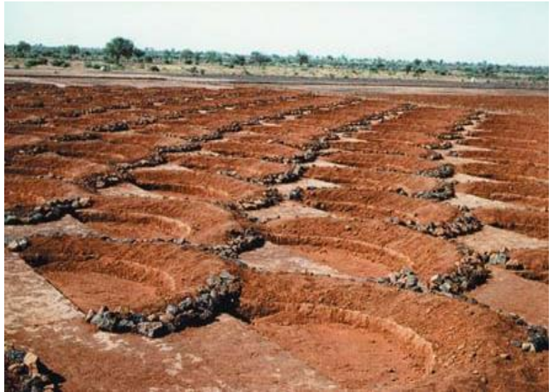
A network of half-moons reinforced with stones and intended to capture and direct limited rainfall
