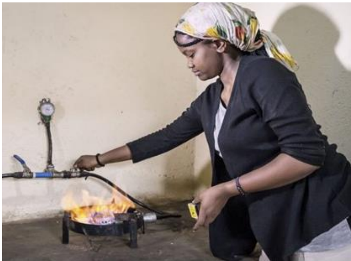
Cooking with biogas generated from farm wastes; note the pressure gauge and valves
