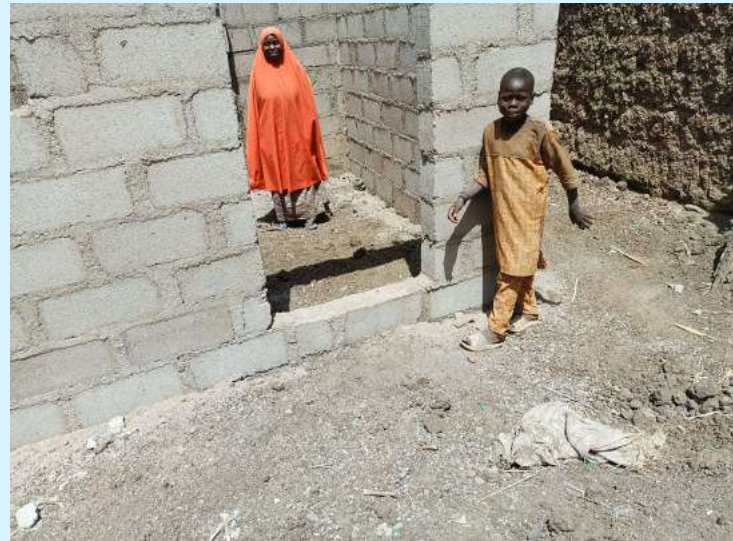
▲ Photo: Mariam Ali' in her new home construction site (Photo Credit FtF-NIAA)
